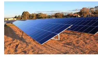
The Visually impressive 468kW ground mount system is expected to produce around 2257kWh/per day saving an estimated 815 tonne of green house gas emissions each year.
